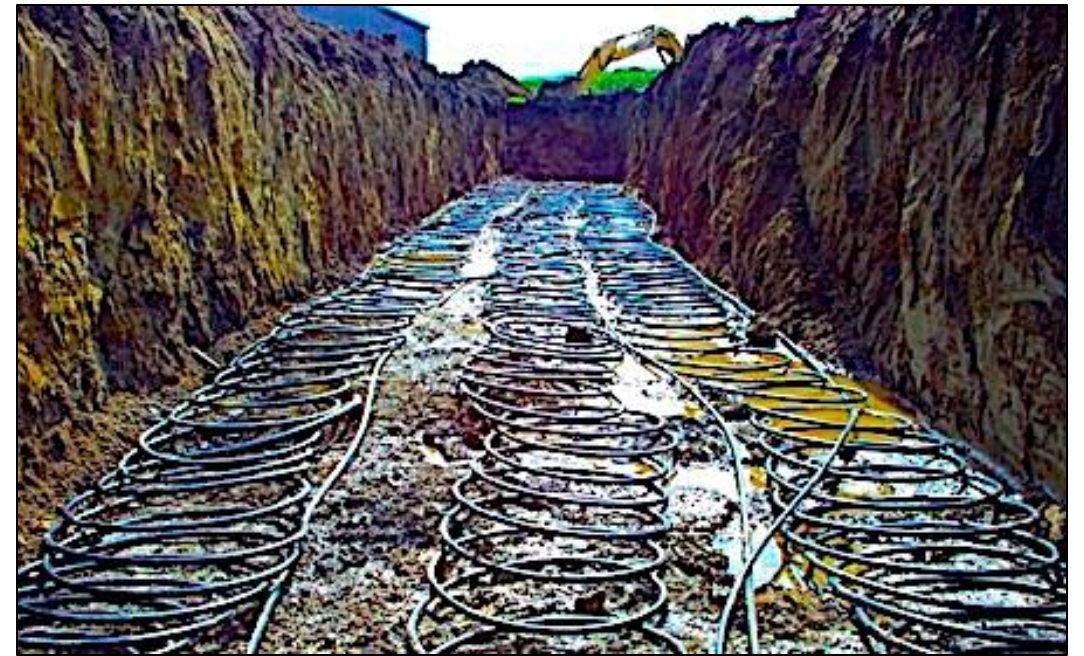
Geothermal heat pump tubing being prepared for burial.
