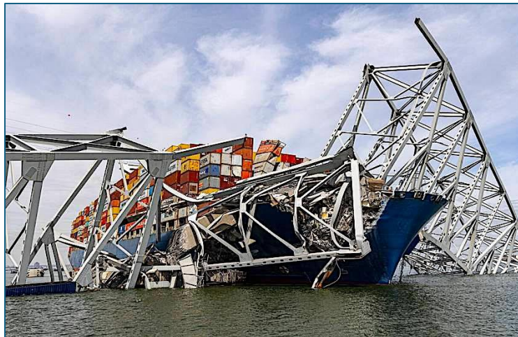
Key Bridge Collapse in Baltimore (3/26/24)
