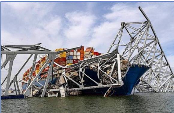
Key Bridge Collapse in Baltimore (3/26/24)
